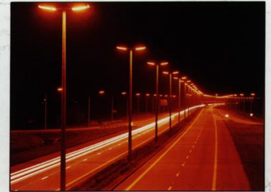
Plate 9 Motorway lighting with low pressure sodium lamps.
